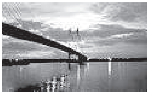
Second Hooghly Bridge(Illuminated)
