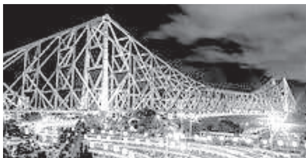
The Illuminated Howrah Bridge
