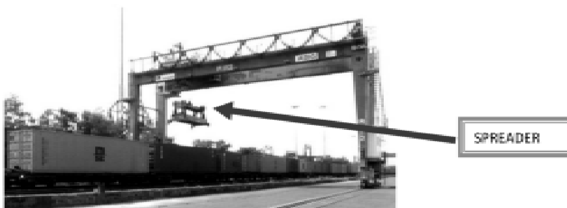
Figure 15 : A Rail-Mounted-Gantry Crane (RMG)
